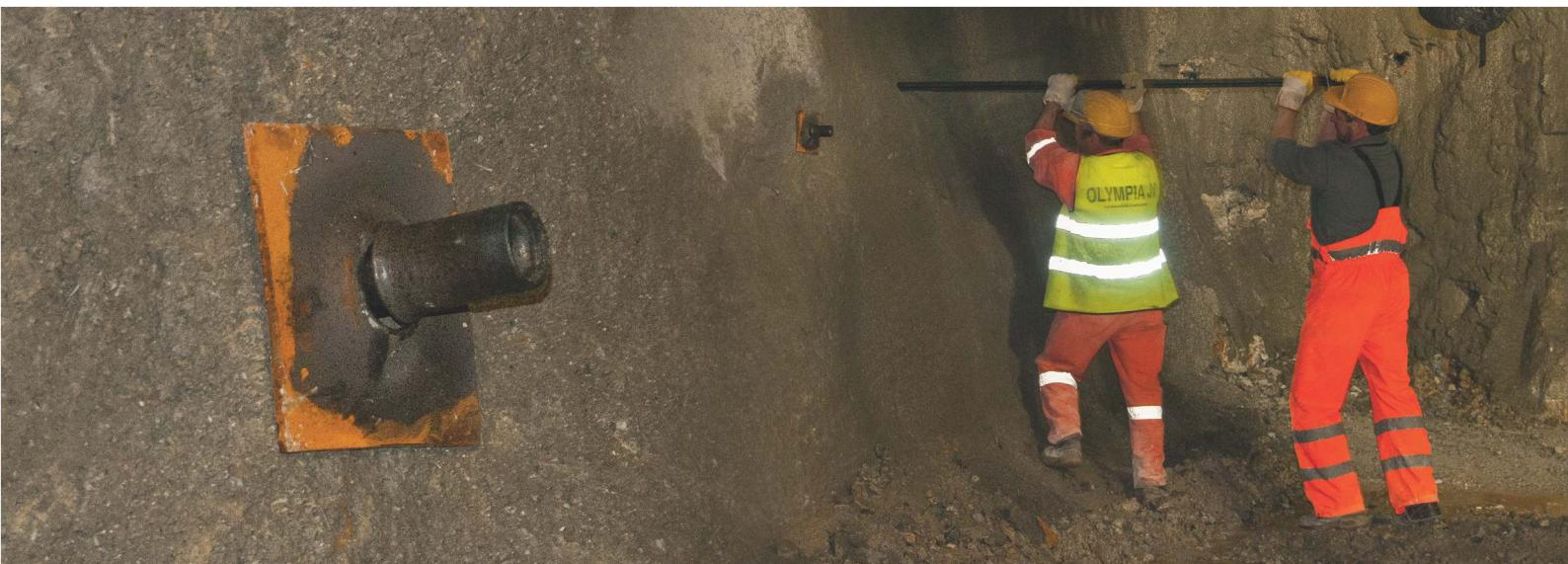
**ELEBOLT™** is a friction stabilizer that is activated by swelling its tubular steel body after the bolt has been inserted in the borehole. Swelling is achieved by injection of high pressure water in the bolt. The swelling action brings the tubular steel body in true and tight contact to the borehole walls thus exerting radial forces to the surrounding rock/strata.
